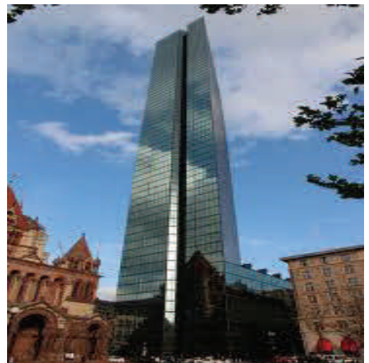
John Hancock Building
